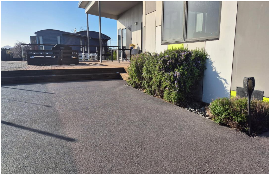
View east to 62 Amaroo Drive from 64 showing part existing deck structure
