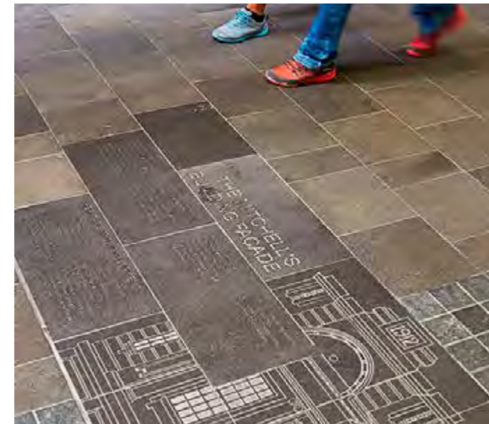
Etched paver wayfinding signage
