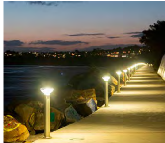
Solar LED bollards will increase ambient lighting at the footpath level to help improve visibility and accessibility
