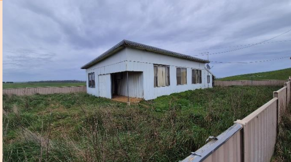
Existing dwelling – Lot 2
