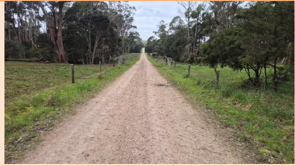
Existing access approximately 200m from Jocks Road – Lot 1 (approx. 4m wide)
