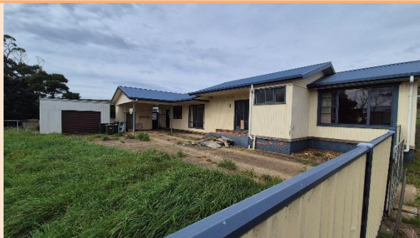
Existing dwelling – Lot 1
