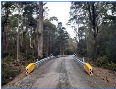
Karl Jaeger Road Bridge
